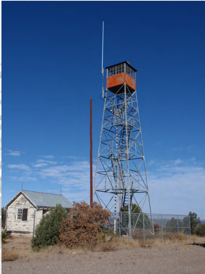
Bluewater Lookout 19 November 2009.
