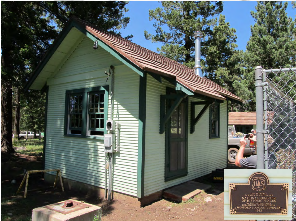
Wofford Complex during restoration in 2014.
