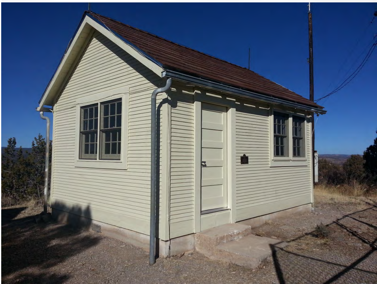
Bluewater Observer's Cabin after restoration 17 January 2014.
